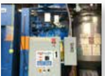
Lower utility costs by tracking gas consumption on individual dryers and making adjustments for inefficiencies
